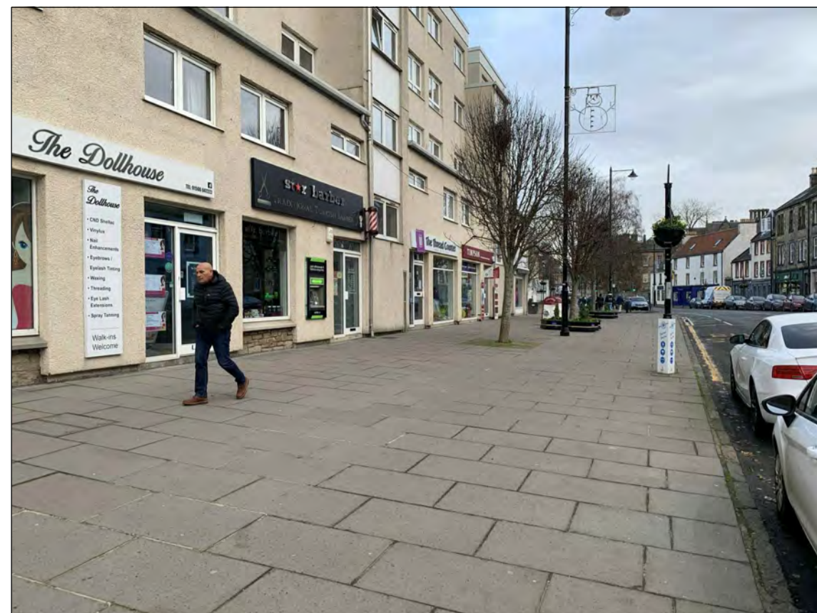
Numbers 9 & 10 Type C - New Whitebeam Trees ( Sorbus aria Lutescens ) proposed into new tree pits
