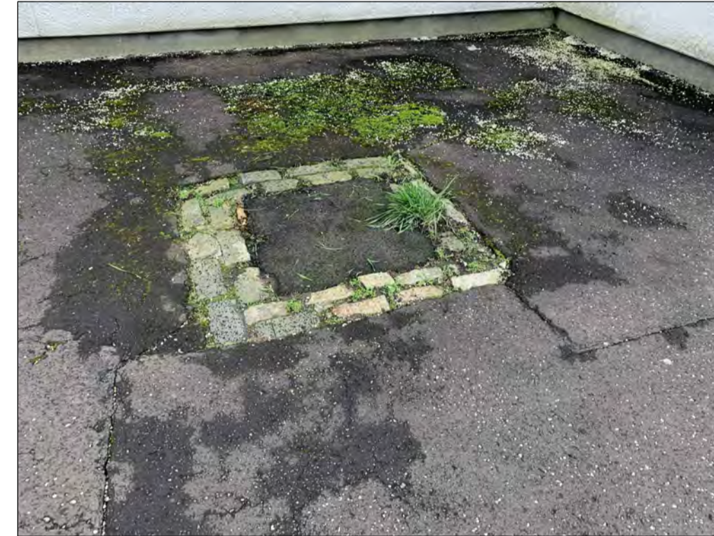
Number 3 - Type B - New Fastigiata Lime Tree ( Tilia cordata 'Green Spire' ) with clear stem to 2m proposed in refurbished Tree Pit
