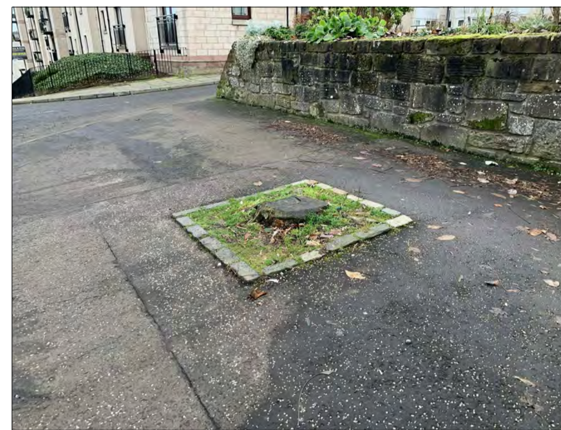
Number 4 - Type B - New Fastigiata Lime Tree ( Tilia cordata 'Green Spire' ) with clear stem to 2m proposed in refurbished Tree Pit
